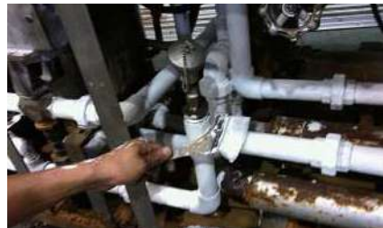
An example of setup for cooling equipment. It prevents corrosion of piping due to condensation.
